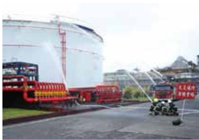
The fire crew set up the water line to sprinkle water
