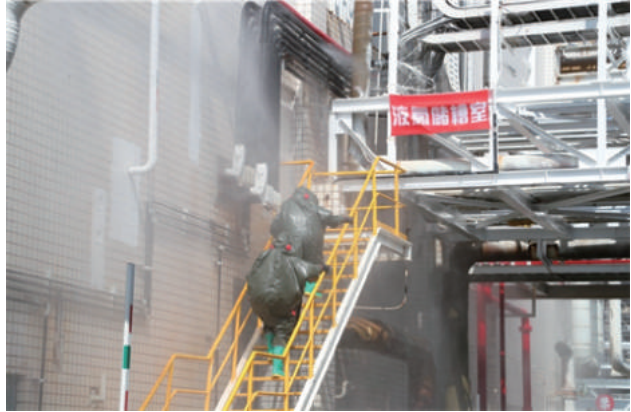
4. The rescue squad enters the liquid chlorine storage tank to stop the leak.
