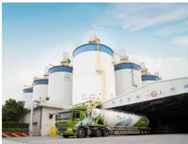
..... Mailiao PVC Plant
