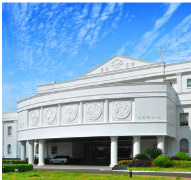
..... Administrative building in Mailiao Industrial Complex
