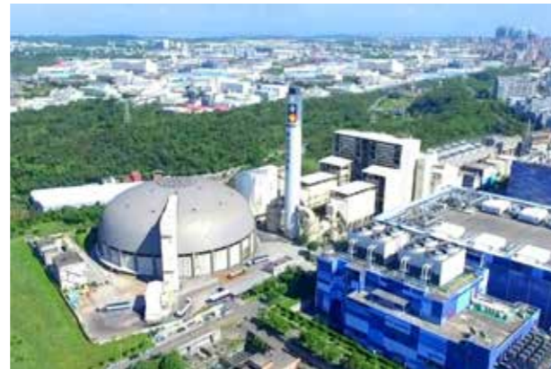
EPC Integration Services For Power Generation
