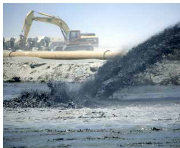
Pumping sand to fill the sea
