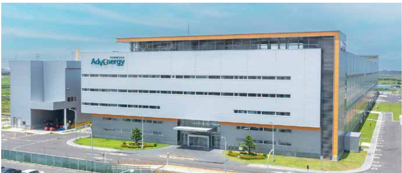
| Taiwan's Largest Battery Cell Manufacturing Facility – Formosa Advanced Technologies' Changbin Plant
