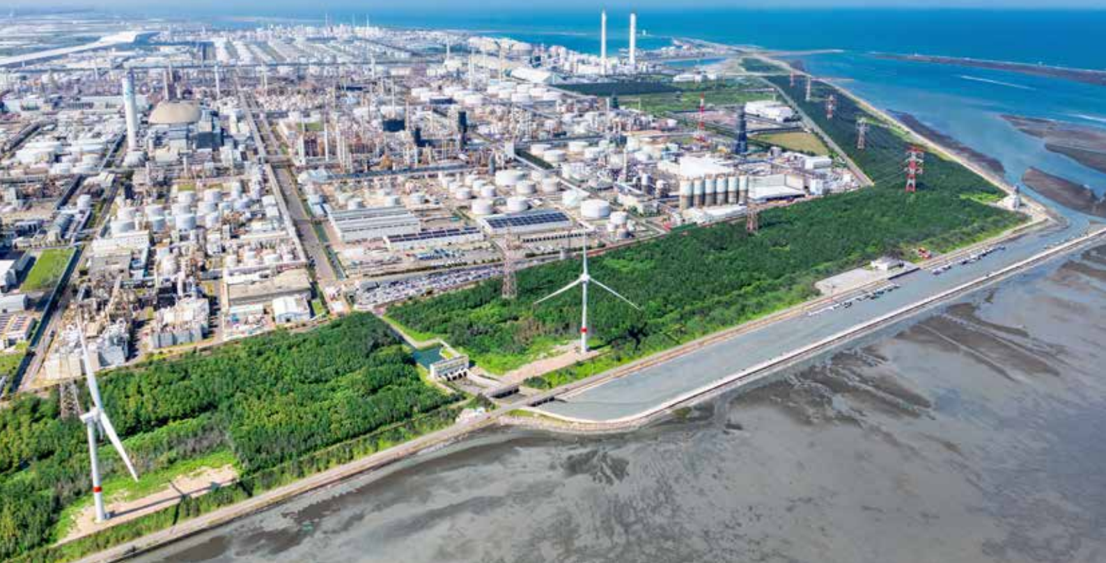
| Mailiao Industrial Complex
