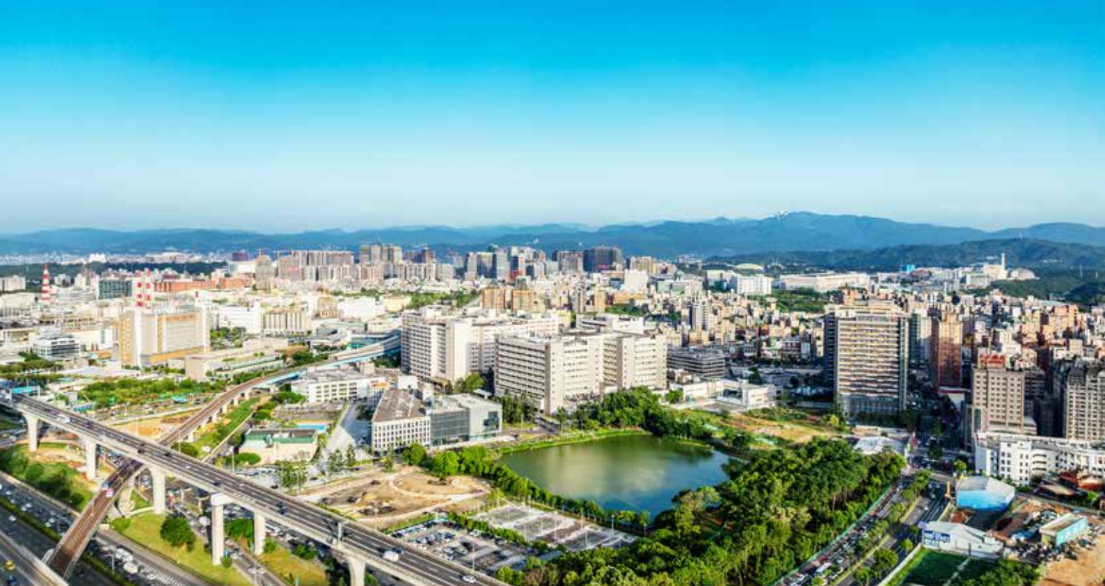
| Aerial View of Linkou Chang Gung Memorial Hospital
