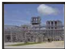
FPC, USA, Point Comfort, Texas
