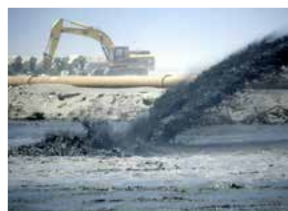
Pumping sand to fill the sea
