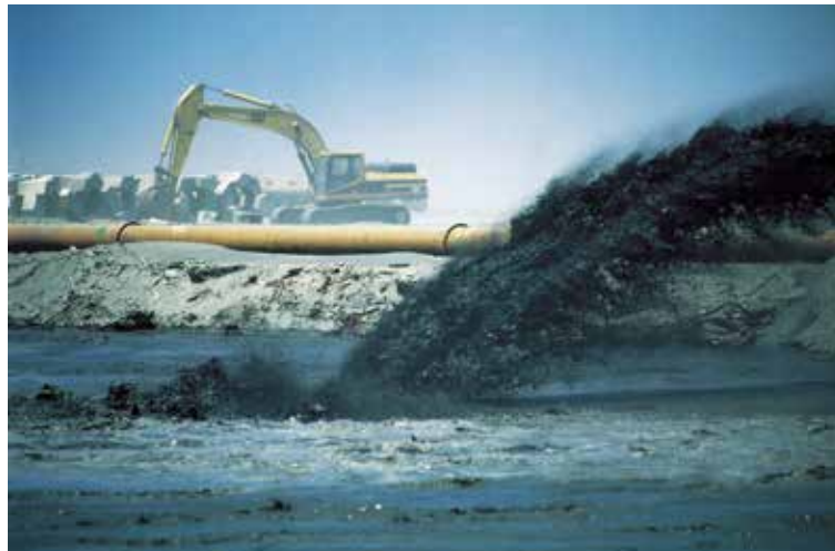
Pipeline end of land reclamation
